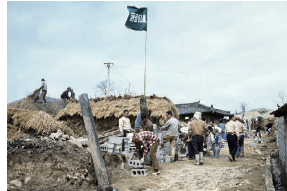
Improvement of thatched roof
